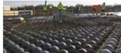
Fig 13 Bubble Deck Slab
