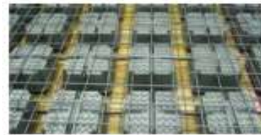
Fig 14 U-Boot Beton Slab
